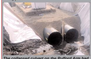
The collapsed culvert on the Rufford Arm had to be replaced with plastic pipes
