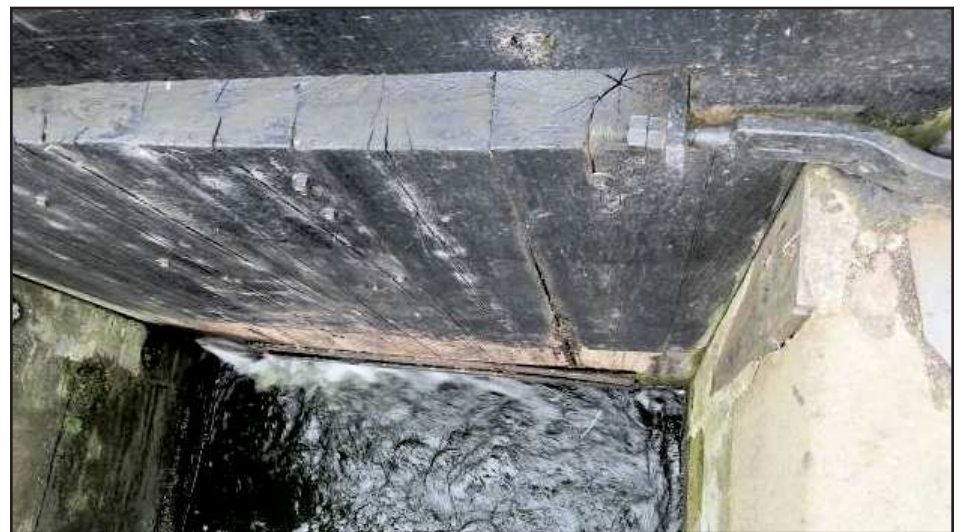
The gate that failed this September causing access issues for local boating festivals as well as boats passing through
