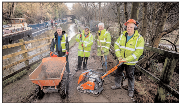
Volunteers at work on the Rochdale's towpath.
