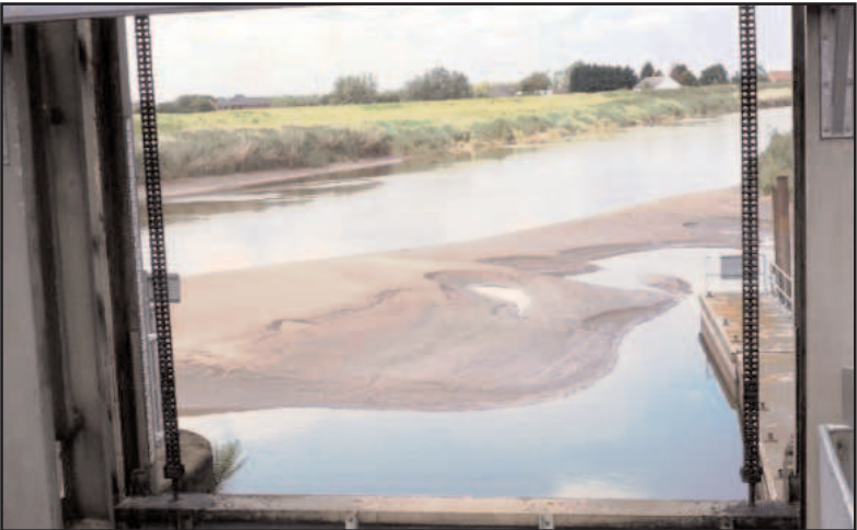
Denver sluice, with the lock on the right, above, and, above right, the silt bank beyond the lock has to be constantly dredged
