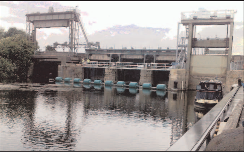
Denver sluice, with the lock on the right, above, and, above right, the silt bank beyond the lock has to be constantly dredged
